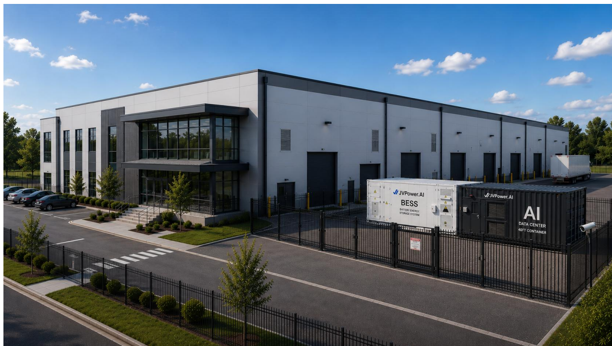
A JVPOWER node on a commercial/industrial site: the AI container plus on-site BESS and dry coolers, beside the host facility.
